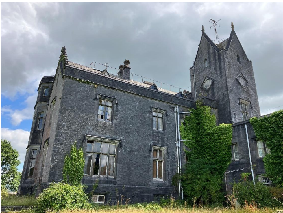
Figure 6 Rear of Mansion © Holland Heritage
