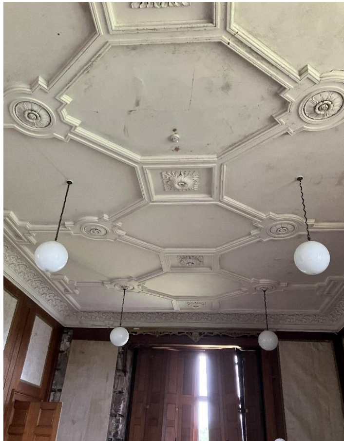
Figure 13 Drawing Room ceiling © Holland Heritage
